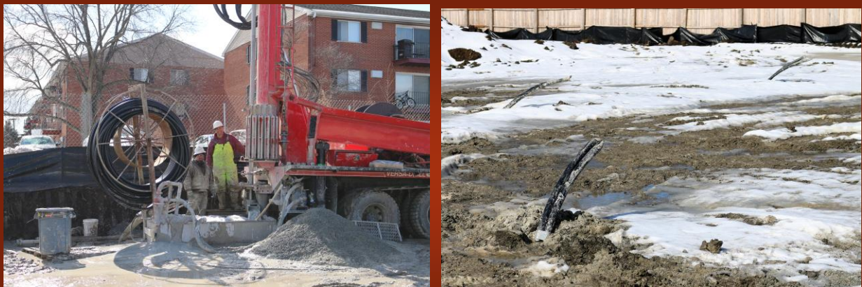
Geothermal wells were drilled 450 feet deep where the earth's temperature is a constant 55°. In the picture on the right you can see the ends of the wells sticking up during the installation process.
