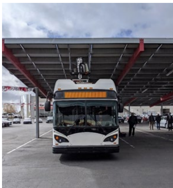
Figure 5. In-Depot Overhead Charging Example (Source: CALSTART)
