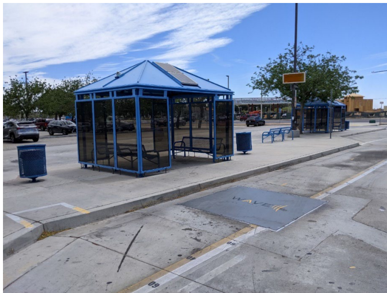
Figure 7. Inductive Charging at Antelope Valley Transit Authority (Source: CALSTART)
