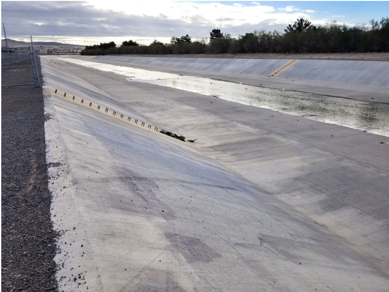
Figure 3. Concrete-lined channel
