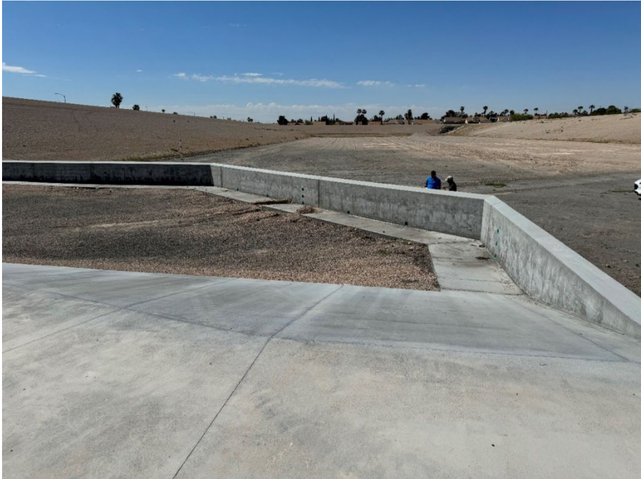
Figure 7. Low-flow feature at Oakey Detention Basin
