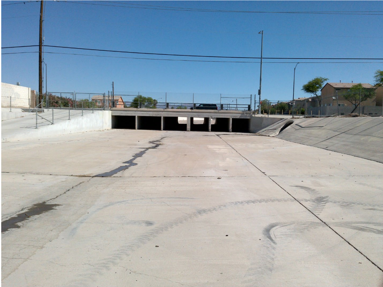
Figure 4. Concrete-lined channel and box culvert
