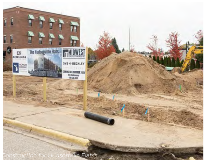
Construction for Hudsonville Flats
