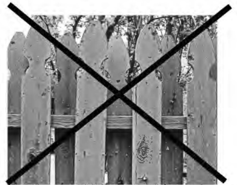
Board on board "shadow-box" fences are not recommended.
