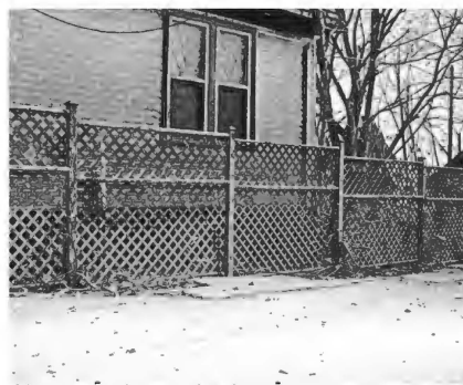
The step down of a fence to accommodate grade change.
