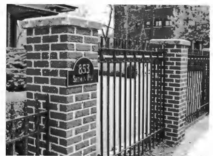
4' to 10' segments between masonry pillars.
