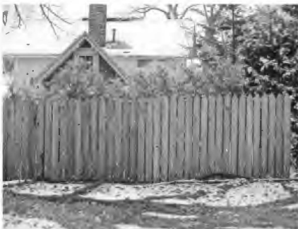
Provide at least the thickness of the board (3/4" - 1") when privacy is a concern.
