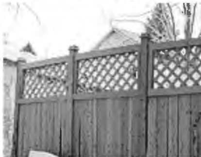
Lattice used as the top of a fence.
