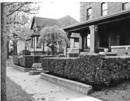
Low retaining wall.
