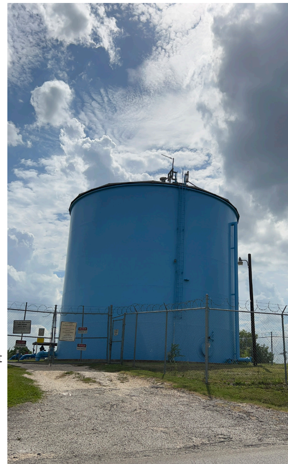
Converse Water Storage Tank
