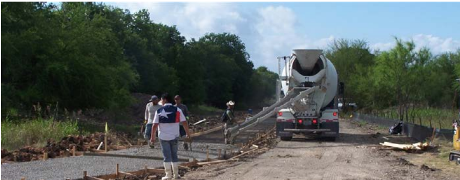
Construction of Greenway Trail System
