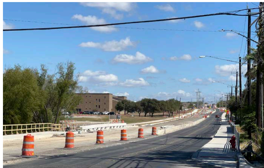
Road Construction on Rocket Lane (Converse, TX)
