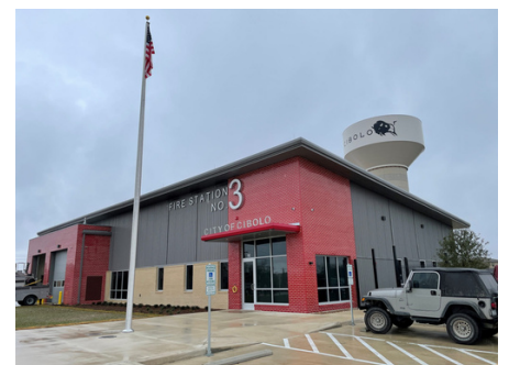
Fire Station #3 1842 Weidner Rd
