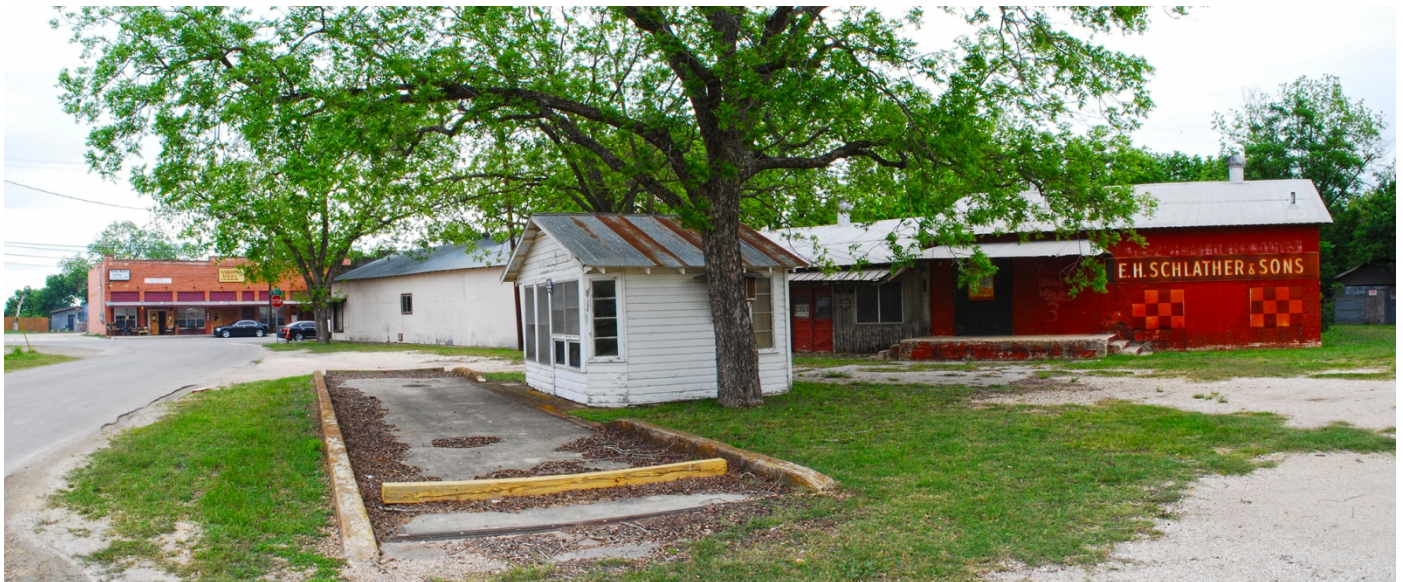
Figure 15: Schlather Feed Store & Weigh Station
