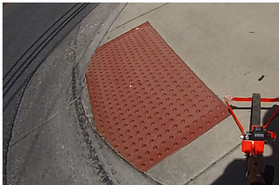
Example of Detectable Warning Surface
