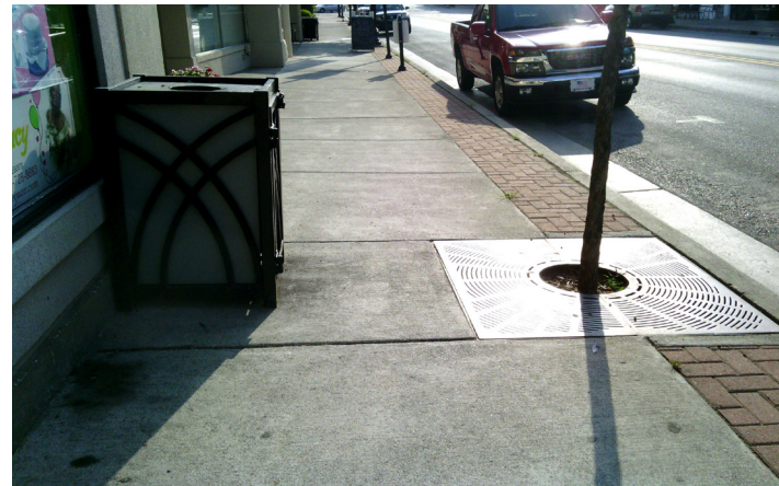
Example of Obstruction
