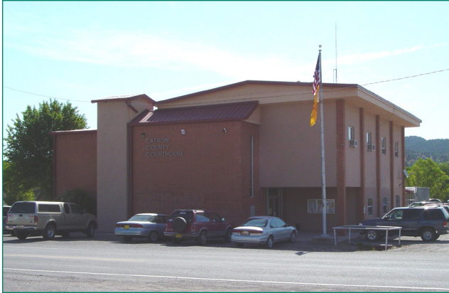
Catron County Building
