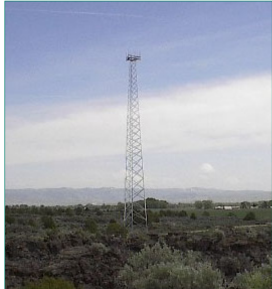
Typical Lattice Cell Tower
