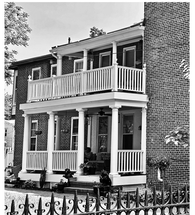
Porch and balcony restoration at 305 East Union Street.
