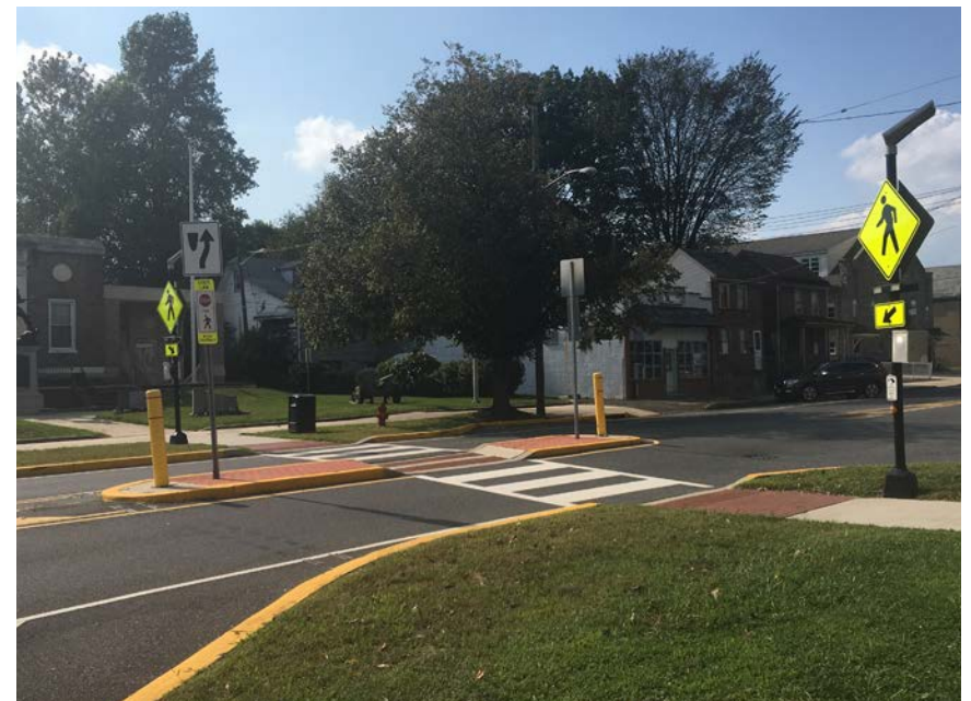
Existing Pedestrian Refuge Island with Rectangular Rapid Flashing Beacon (RRFB) near Wilbur Watts Elementary School
