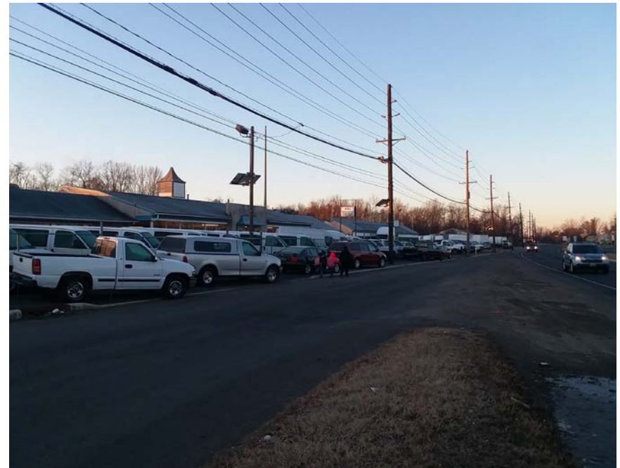
Missing Pedestrian Connection at US 130 near Logan Ave
