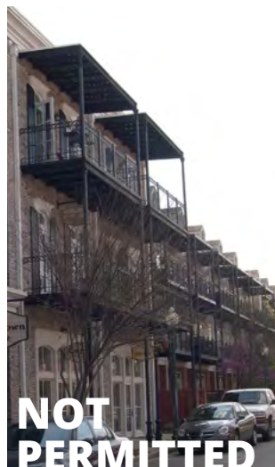
Balconies: Covers More than 40 Percent of Facade
