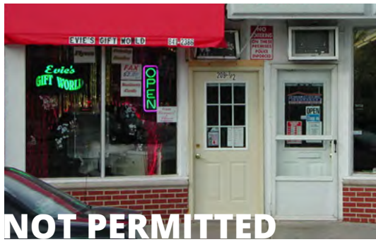
Residential Grade Doors on Commercial Buildings.
