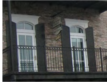
Appropriately Scaled Shutters.
