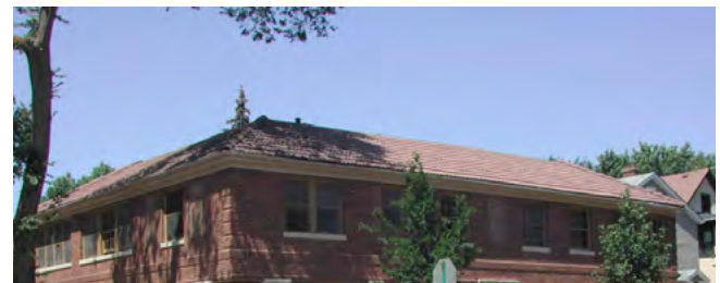
Roof Materials: Ceramic Tile
