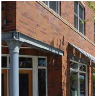
Brick with Metal Details
