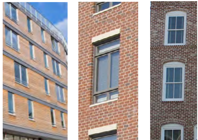
Figure 62-217-4. Vertically Oriented Windows with Expressed Lintels
