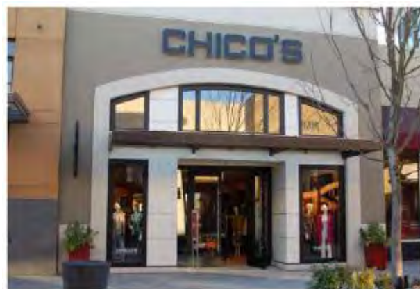
Commercial Grade Doors & Windows on Commercial Buildings.
