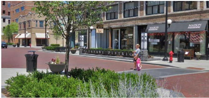
Curb bump-outs with landscaping can shorten crosswalk distance and improve the area's visual appeal.
