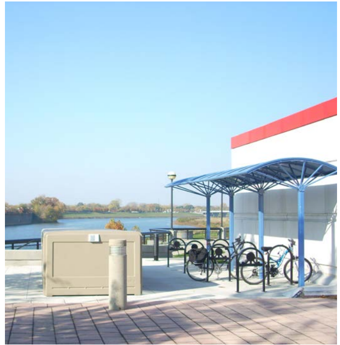
Example of a sheltered bike parking with secured bike storage facilities.
