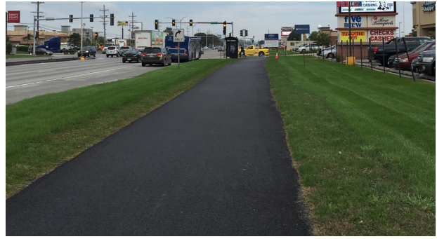
Newly built sidepath on North Ave through Melrose Park
