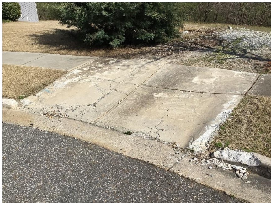
Figure 6.15 1841-1845 Madrid Falls Street View
