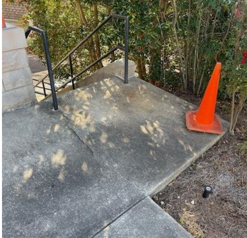
Figure 8.4 4983 Highway 53 – Stair Landing
