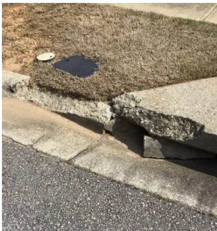
Figure 6.16 1600 Sahale Falls Drive Street View – Left of Catch Basin
