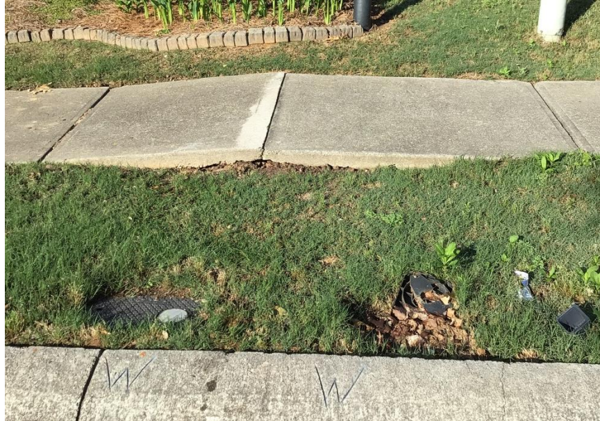
Figure 2.1 5904 838 New Liberty Way Street View
