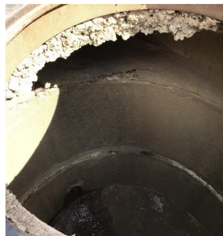
Figure 6.18 1600 Sahale Falls Drive – Interior View of Structure
