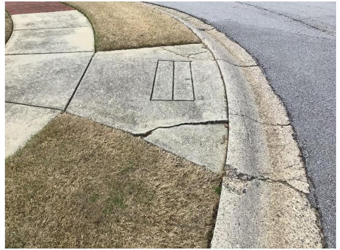
Figure 6.6 Fisk Falls Drive and Madrid Falls Drive Intersection Southwest Street View
