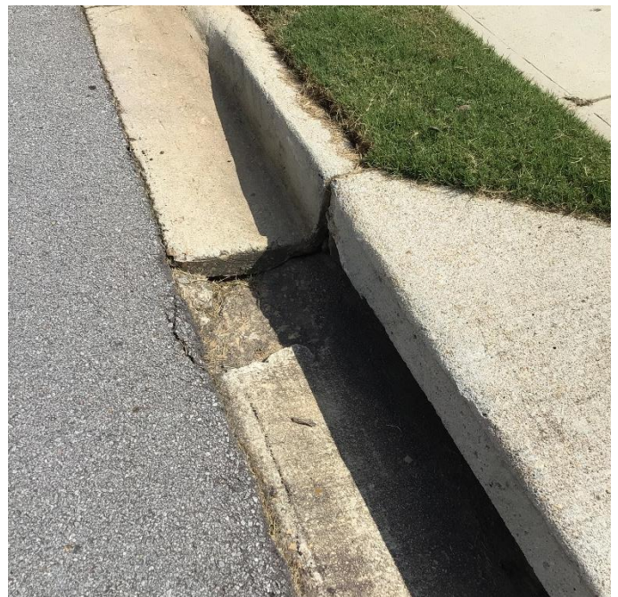
Figure 3.12 7370 Silk Tree Pointe – Curb and Gutter
