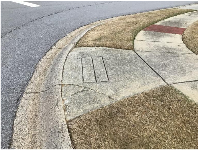
Figure 6.5 Fisk Falls Drive and Madrid Falls Drive Intersection Northeast Street View
