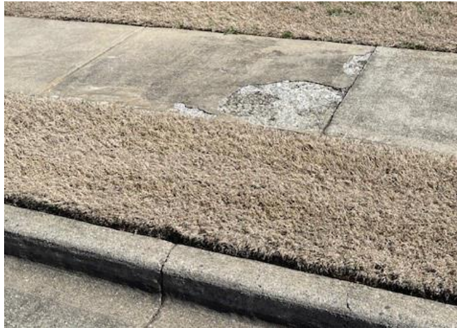
Figure 1.4 2437 Commissioner Cove Street View
