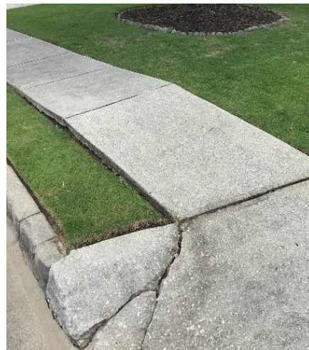
Figure 5.4 5767 Berkshire Trace – Raised Sidewalk
