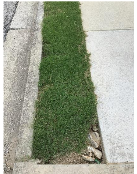
Figure 5.15 6225-6229 Riverview Parkway – Voids
