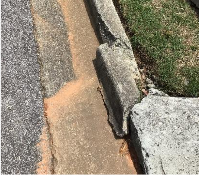
Figure 5.1 5735 Berkshire Trace – Curb and Gutter
