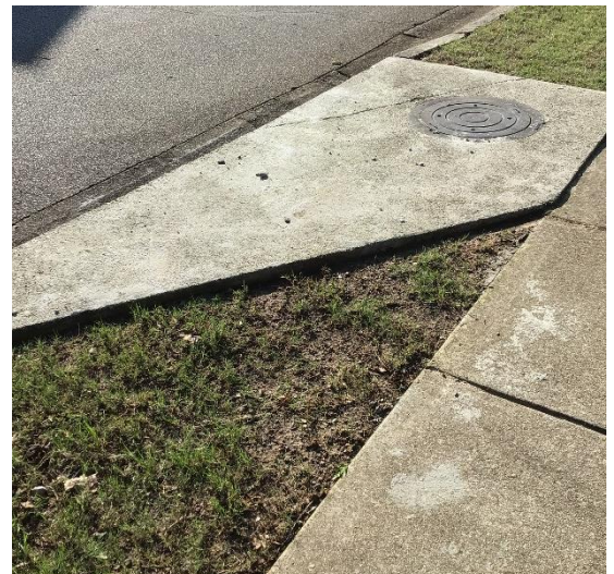
Figure 2.3 852 New Liberty Way – Area to be Backfilled
