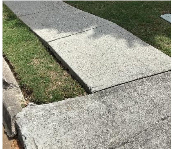
Figure 5.2 5735 Berkshire Trace – Sidewalk
