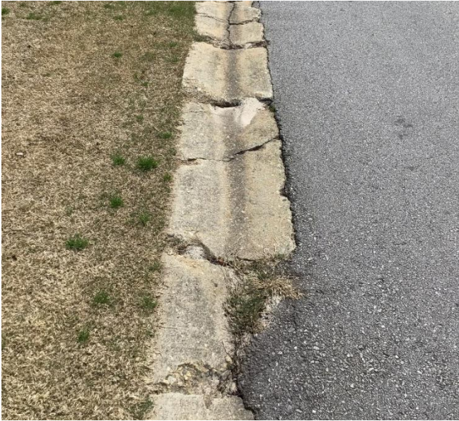
Figure 6.1 Fisk Falls Drive South Street View
