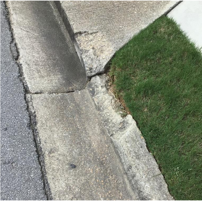
Figure 3.13 7371 Silk Tree Pointe – Curb and Gutter
