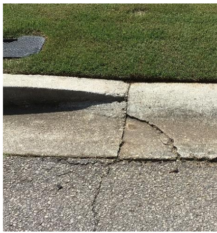
Figure 6.17 1600 Sahale Falls Drive Street View – Right of Catch Basin
