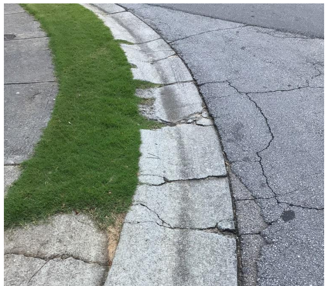
Figure 3.5 Grand Hickory Drive at Bald Cypress Drive – Curb and Gutter
