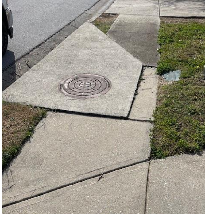
Figure 3.1 2641 Bald Cypress Drive
