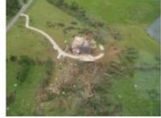
Damage to home on Old Cedartown Road just south of Lindale (Floyd County)
