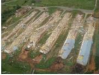
Chicken houses destroyed on Mountain Home Road (Polk/Floyd County line)
