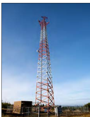
SELF-SUPPORTED LATTICE TOWER
