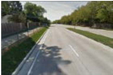
A sidepath along a portion of N. Arlington Heights Rd., in Buffalo Grove, near Buffalo Grove High School, helps protect bicyclists and pedestrians from the heavy traffic.
