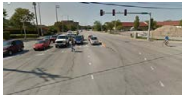
Large arterial crossing with inadequate accommodation for pedestrians or bicyclists (Algonquin and Arlington Heights Roads).
