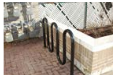
"Wave" style rack installed in manner that severely limits its use
