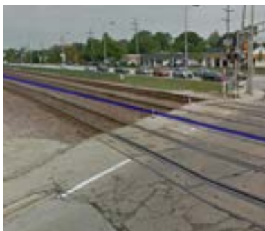
Looking north over the rail line just south of the intersection of Wilke Road and Northwest Highway.
