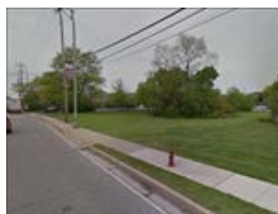
Obstructions in sidewalk (Arlington Heights Road)
