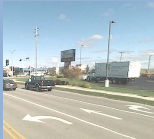
Figure 8: S Kensington Dr is an example of a street that may require reconstruction to accommodate bikes.
