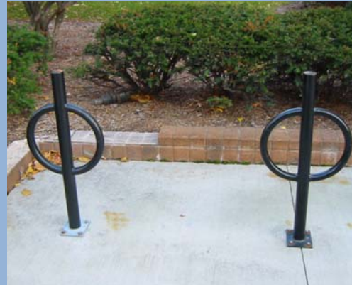
Figure 6: Racks are mounted incorrectly near Houdini Plaza (rotate 45 degrees)
