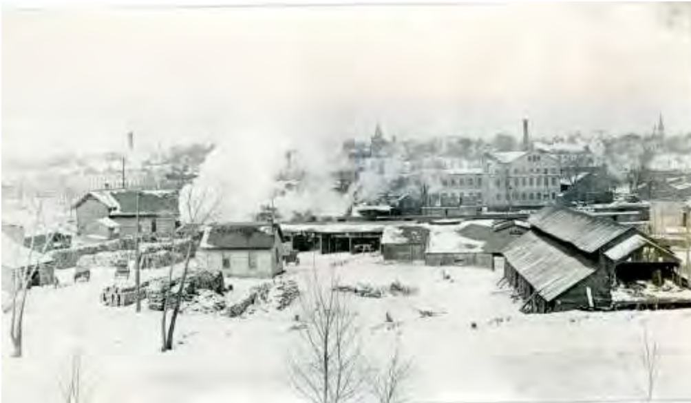
Image L: South façade viewed from across river, undated. (Courtesy of: Appleton Public Library, PP-4-8)
