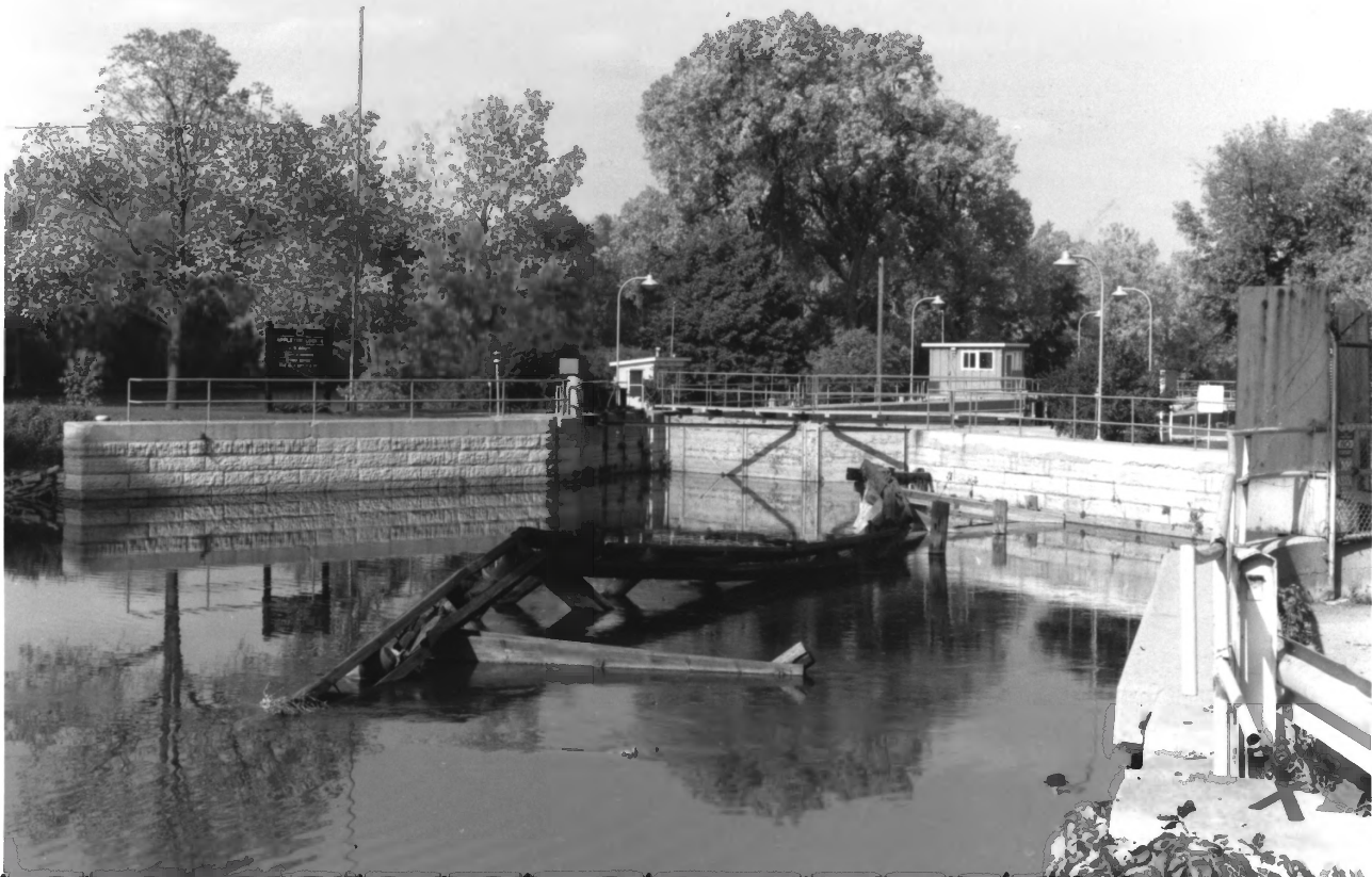
Appleton Lock & Dam Dist, Appleton, Outagamie County, Photo # 1 of 2
