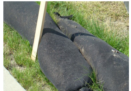
Overlap ends of two sections. The stakes at this site should have been driven into the practices or the teepee method could have been used.
