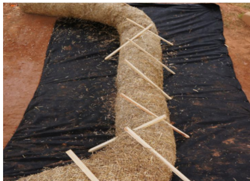
Stakes can be driven into the center or the teepee method can be used. Blankets can be used beneath both practices to reduce scouring.
