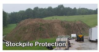
Issue: Exposed soils with rill erosion on stockpile.
