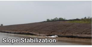
Issue: Rill erosion, overwhelmed silt fence.
