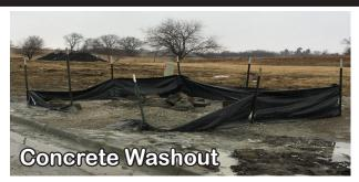
Issue: Silt fence damaged, no liner, exposed access, accumulated washout and solids.
