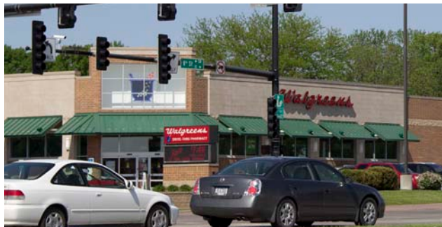
Top: Old Town provides community services such as a barber shop. Above: Walgreens primarily serves nearby residents.
