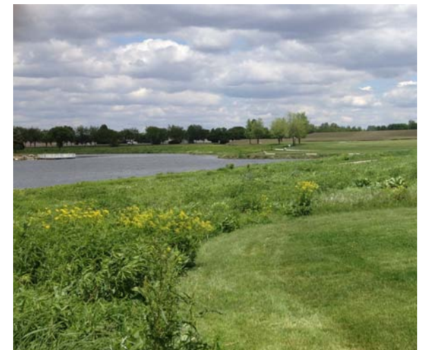
Above: A stormwater detention pond with a native vegetation buffer can manage stormwater and provide an amenity.
