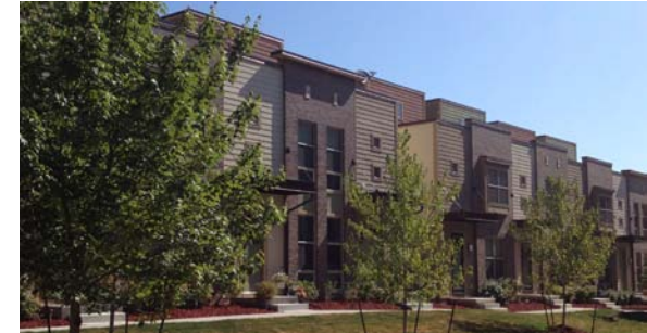
Row-houses with rear garage (Des Moines)
