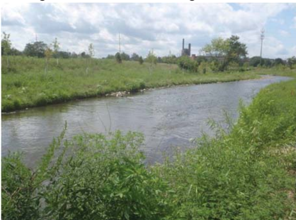
Figure 5. ST 10+00 looking downstream
