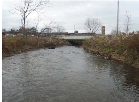
Figure 6. ST 12+00 looking downstream
