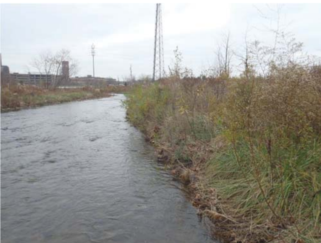
Figure 3. ST 6+00 looking downstream
