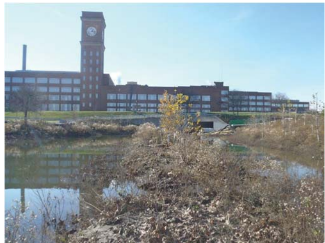
Figure 12. ST 24+00 looking downstream
