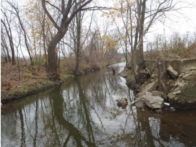
Figure 1. ST 2+00 looking downstream
