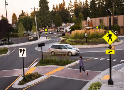
RRFB AT ROUNDABOUT INTERSECTION
