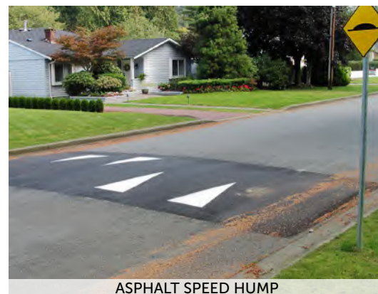
ASPHALT SPEED HUMP
