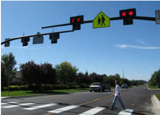
PEDESTRIAN HYBRID BEACON AT CROSSWALK
