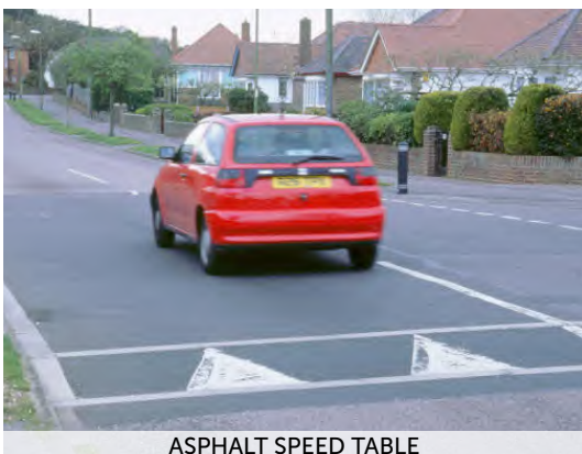
ASPHALT SPEED TABLE
