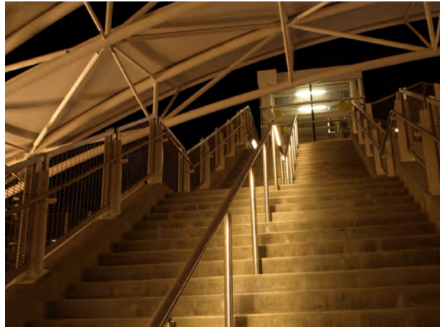
Figure 5.41 Appropriate Stair Lighting. Copyright: Clanton & Associates, Inc.
