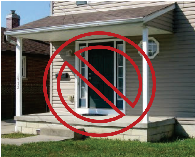
Small porch columns and a lack of railing discourages residents from using the porch.
