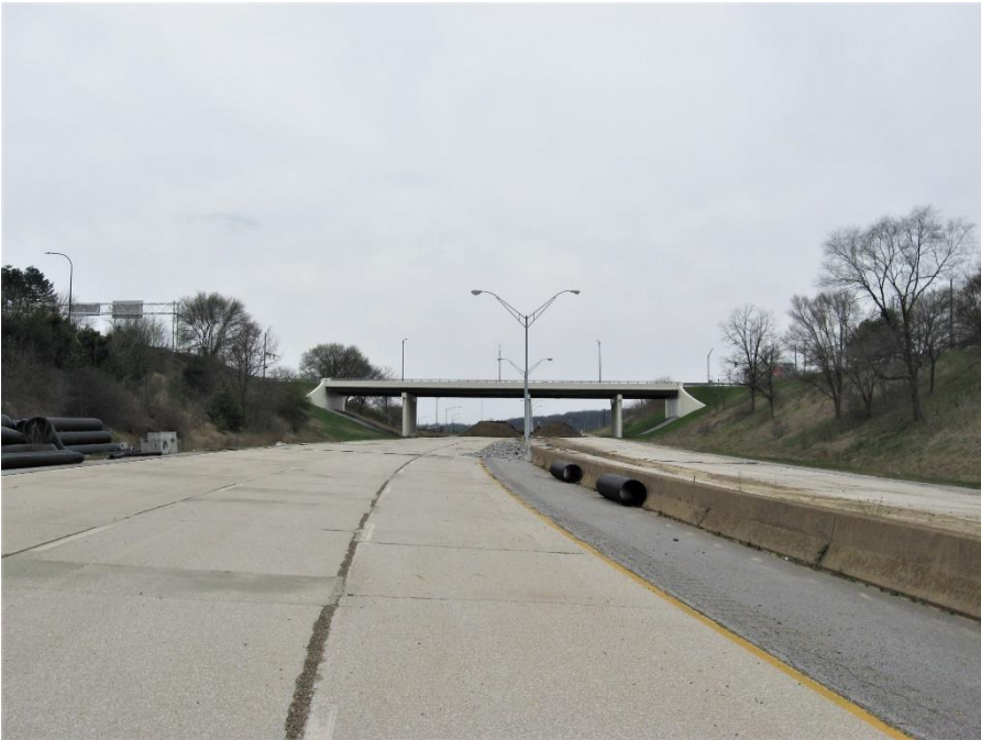
Innerbelt view south towards Center St. Bridge
