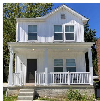
Recent market-rate development along Rhodes Ave. demonstrates the demand for infill housing development
