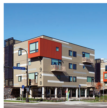
Future infill housing can leverage “missing middle” types like duplexes and small walk-up apartments to meet more diverse housing needs.
