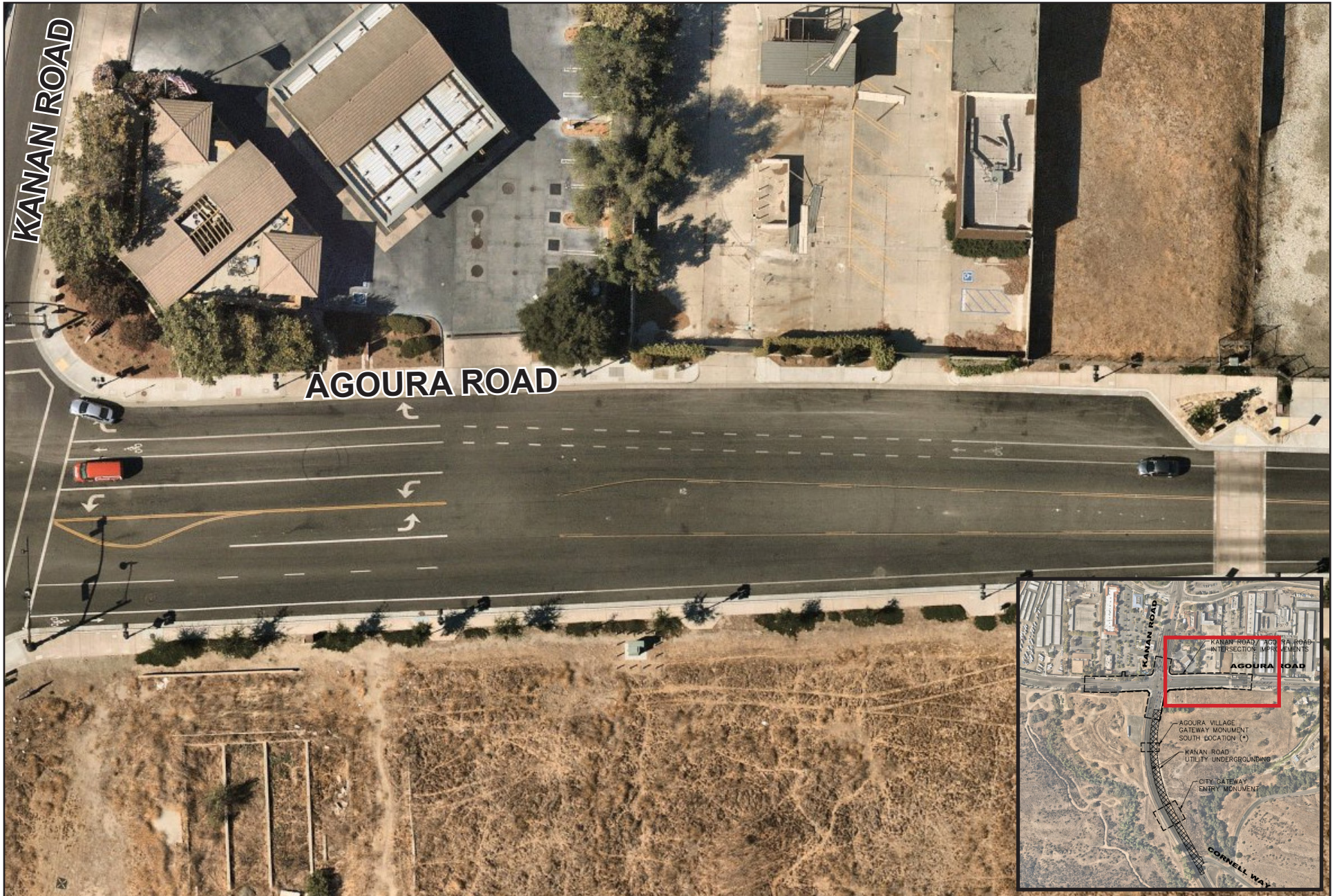
FIGURE 3C: EXISTING KANAN ROAD/AGOURA ROAD INTERSECTION (EAST LEG)
