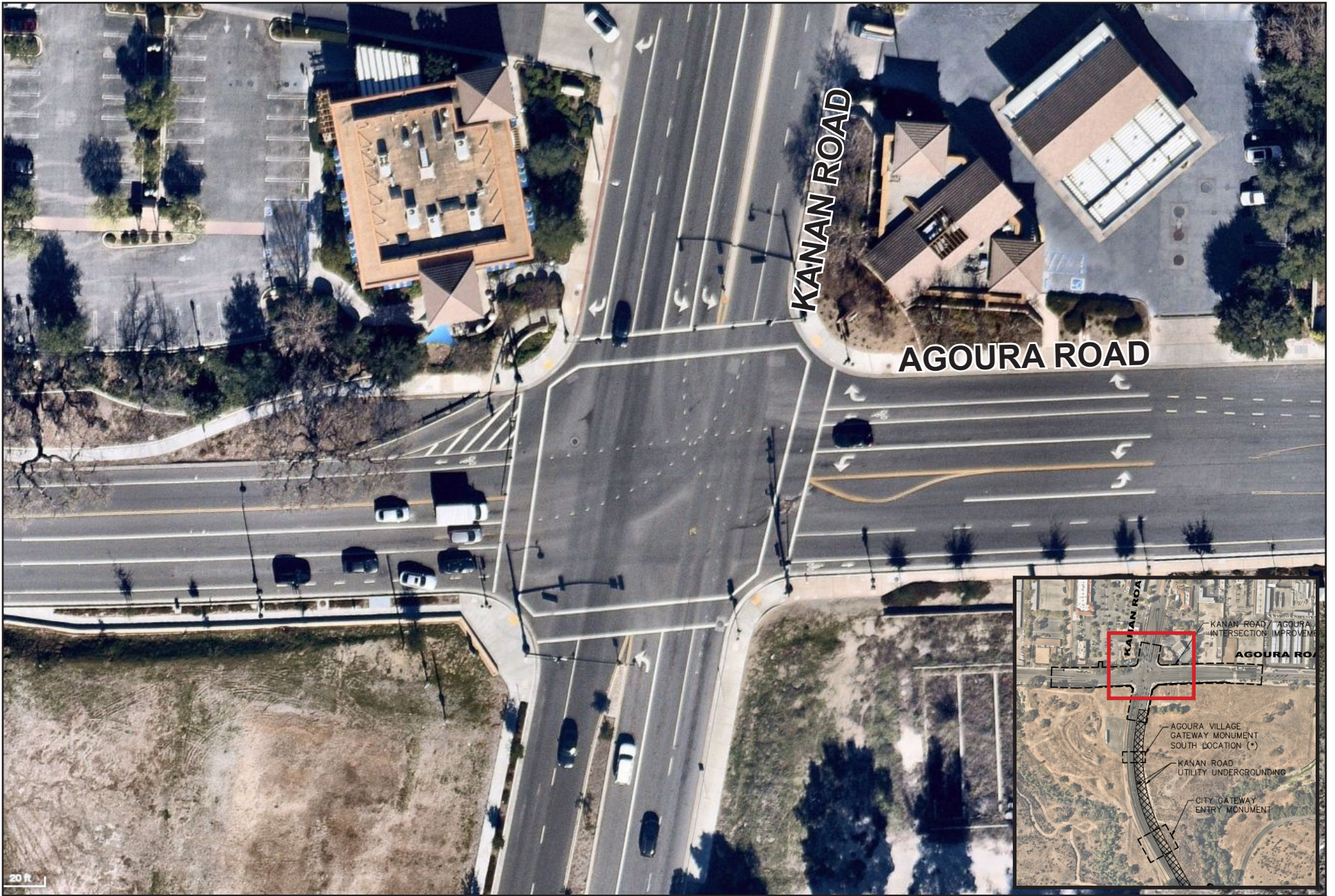
FIGURE 3: EXISTING KANAN ROAD/AGOURA ROAD INTERSECTION (NORTH LEG) Kanan Road/Agoura Road Ultimate Intersection Improvements Project
