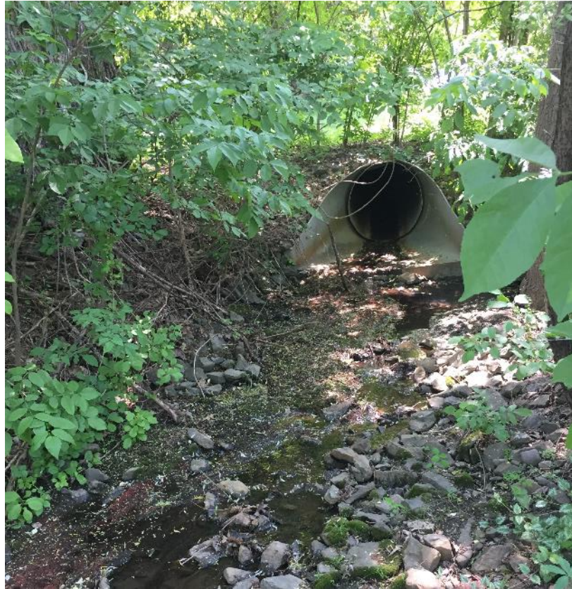
View of the discharge of the 42" dia. closed pipe storm sewer main near Denise Dr. (see red dot in the image to the right)
