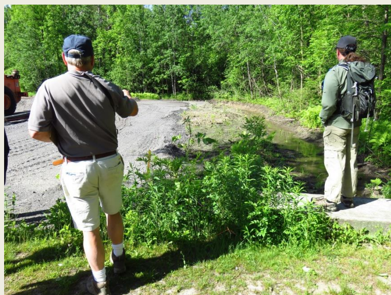
Fill next to edge of wetland
