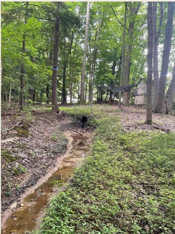
Stormwater culvert discharge
