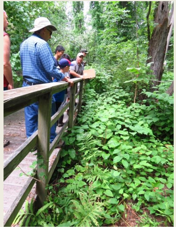
Footbridges need clearing and maintenance
