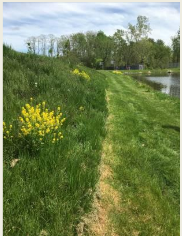
Steep embankment where grass is allowed to grow
