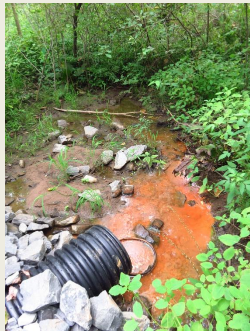
Effluent from neighbor's yard
