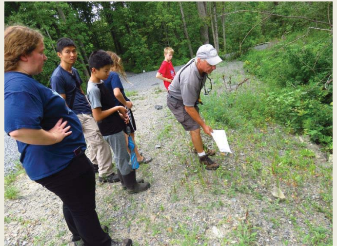
Gravel fill has washed into wetland that can be restored
