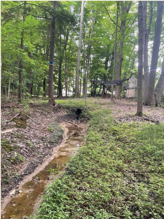
Stormwater culvert discharge
