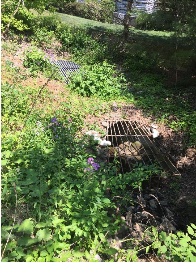
View of both storm water entry grates at the transition from grade level open creek flow to closed pipe near backyard of 1435 Rosehill Blvd.
