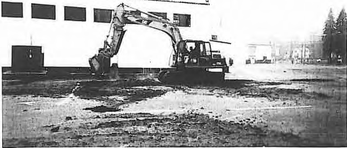
BEGINNING OF EXCAVATION ON ROW 1
