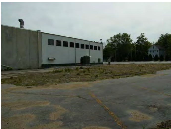
View of the driveway/parking area north of the main facility where the leather remediation project was completed.
