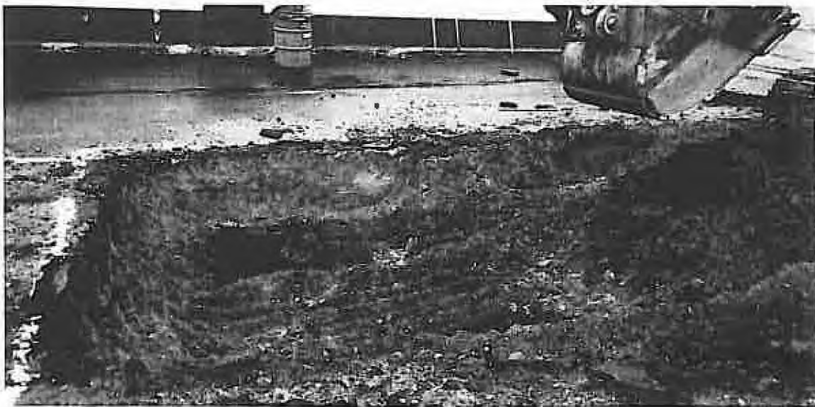
REMOVAL OF FILL SOIL ON ROW 1
