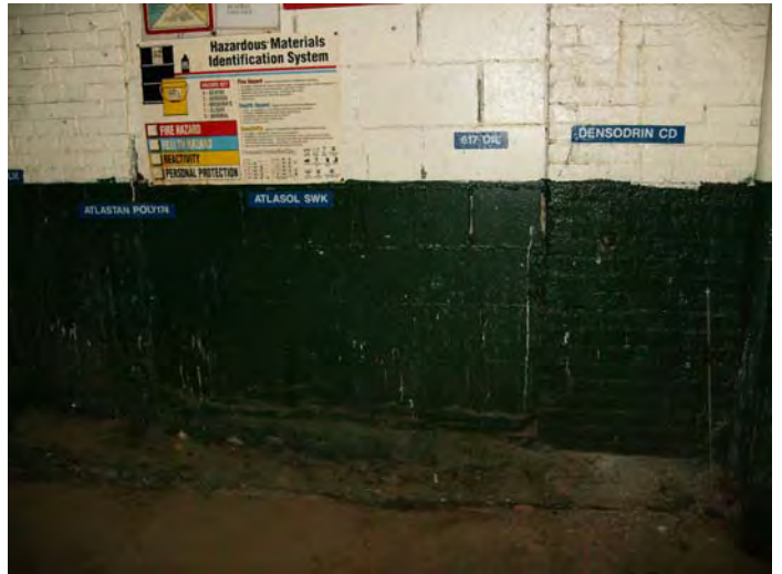
View of the wet weigh up and drum storage area.
