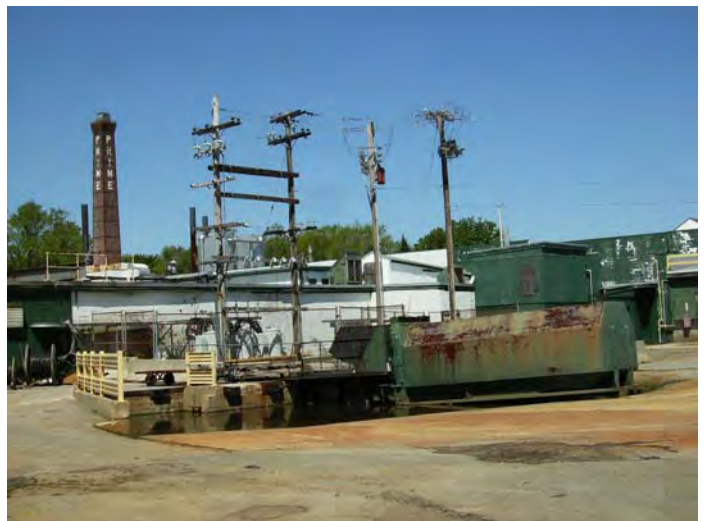
View of the loading dock area east of the main facility building. Standing water was observed.
